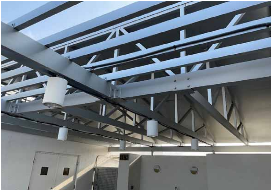
Roof Terrace Shelter
