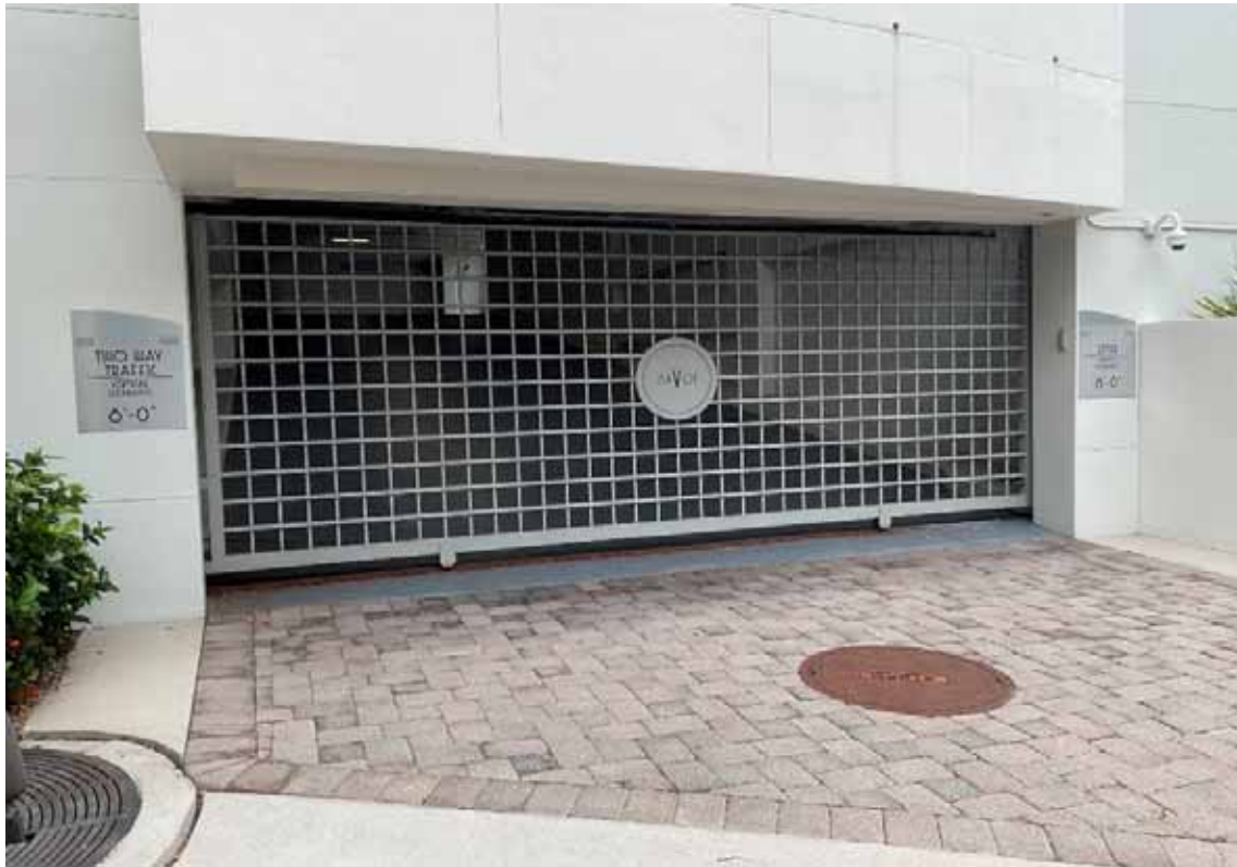
Garage Gate - North
