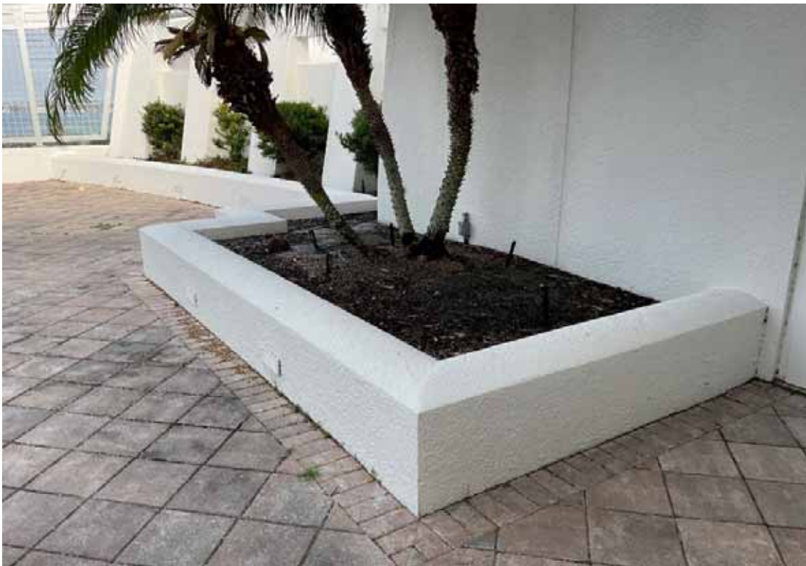
Roof Terrace Planter
