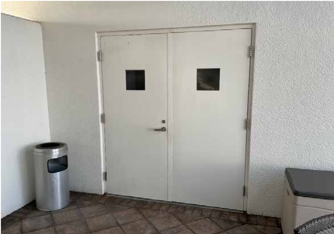
Doors - Roof Terrace
