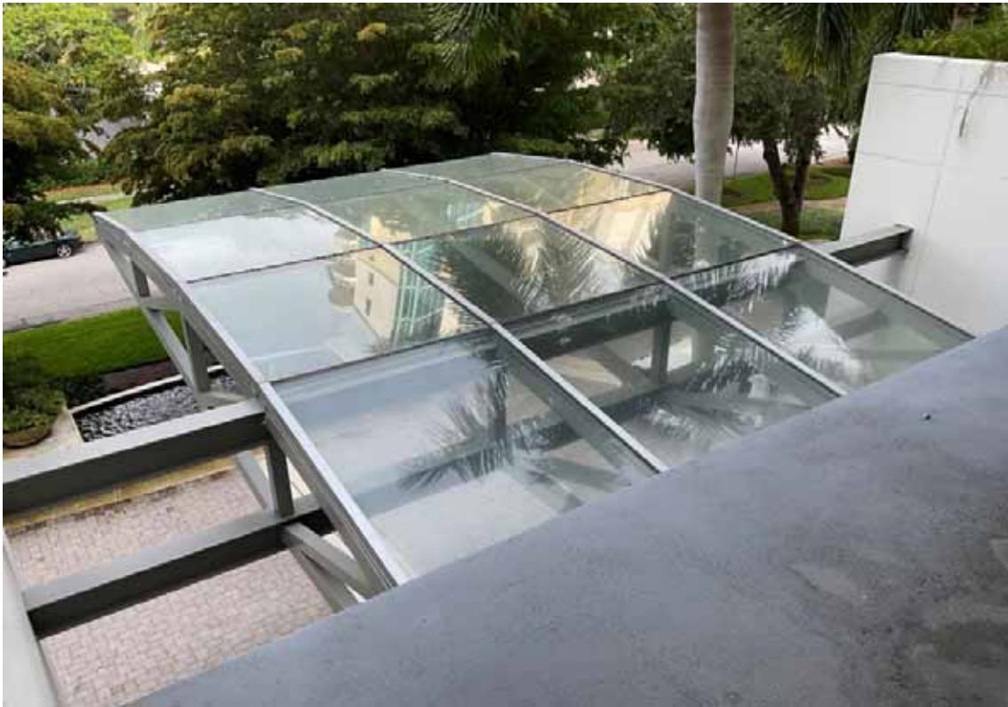
Covered Entry Roof
