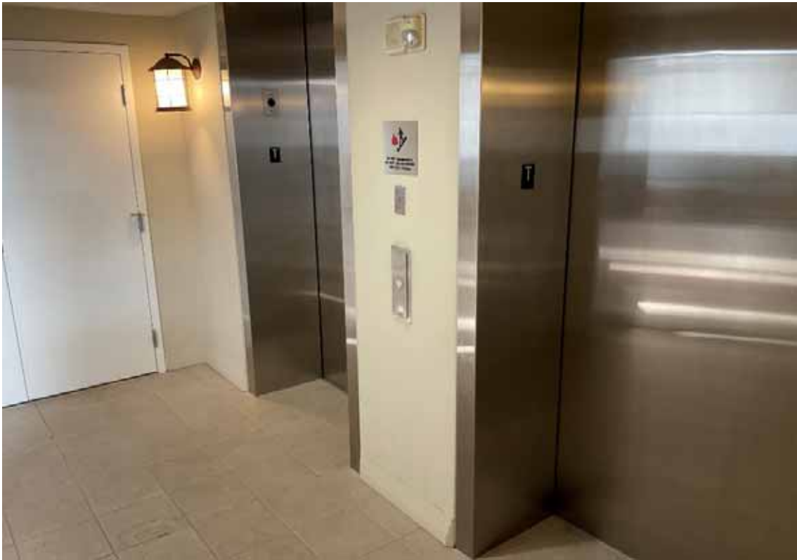
Roof Terrace Elevator Lobby
