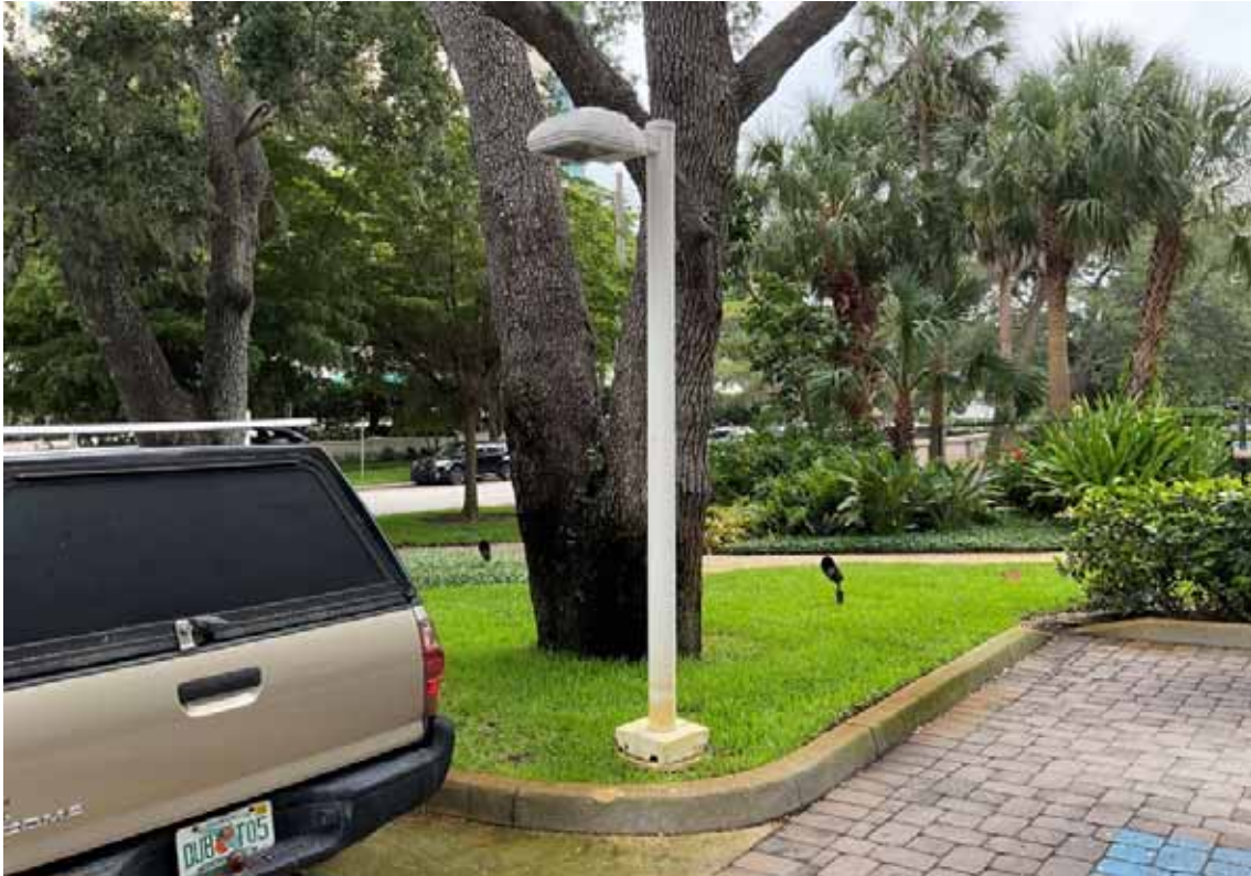
Light Pole & Fixture - Driveway
