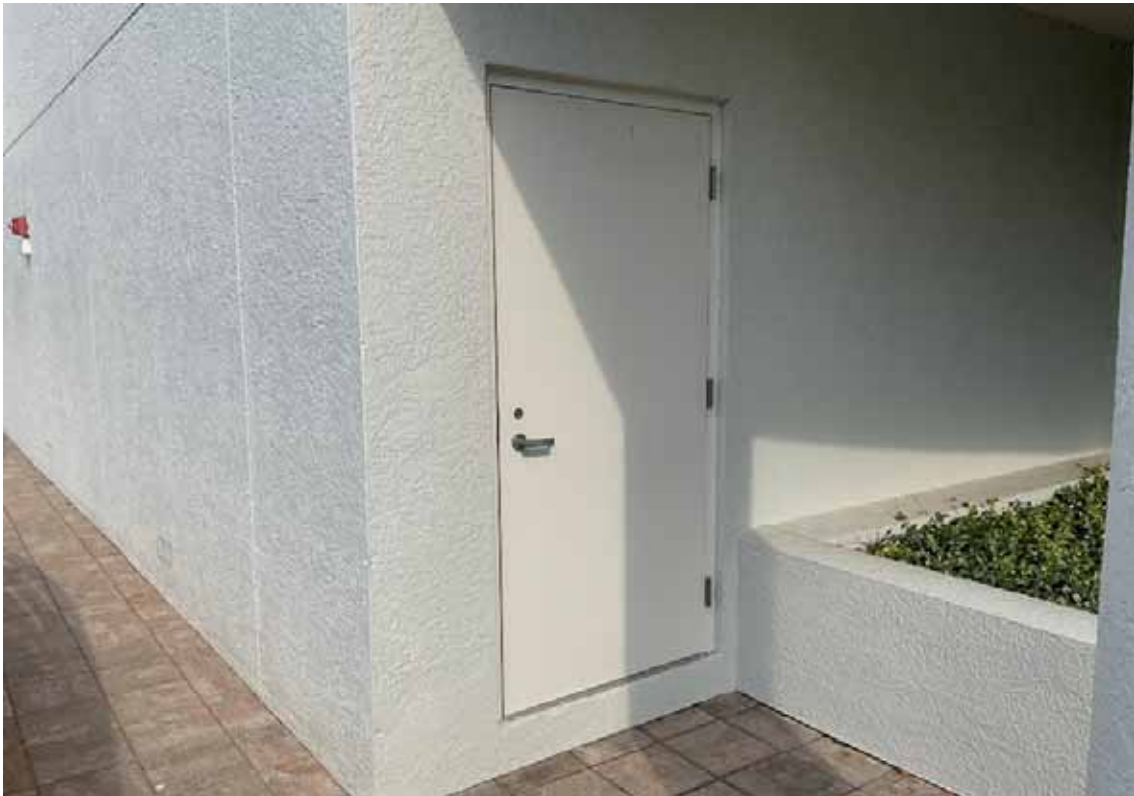
Door - Mechanical Room
