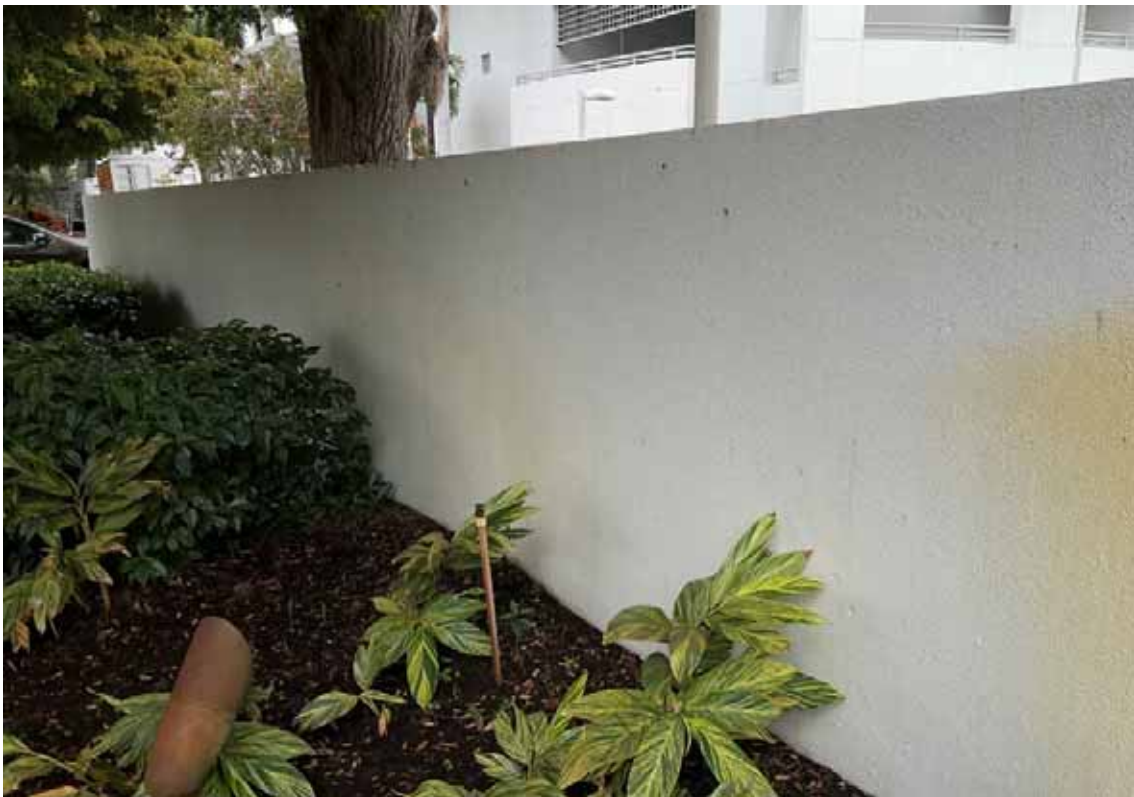
Site Wall - Property Line
