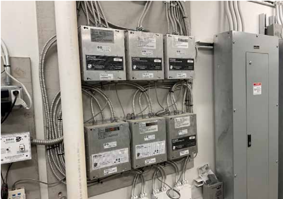
Low Voltage Lighting Control
