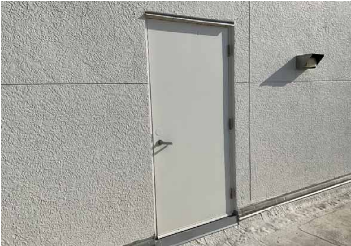
Door - Roof Access
