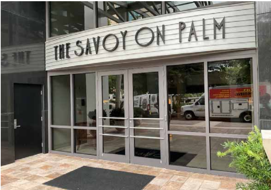
Windows and Doors - Lobby
