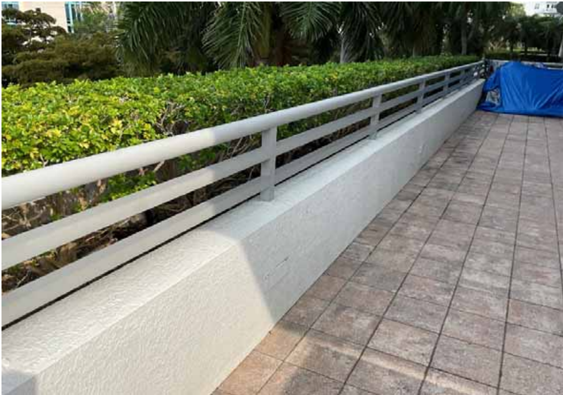
Level 3 Terrace Railing
