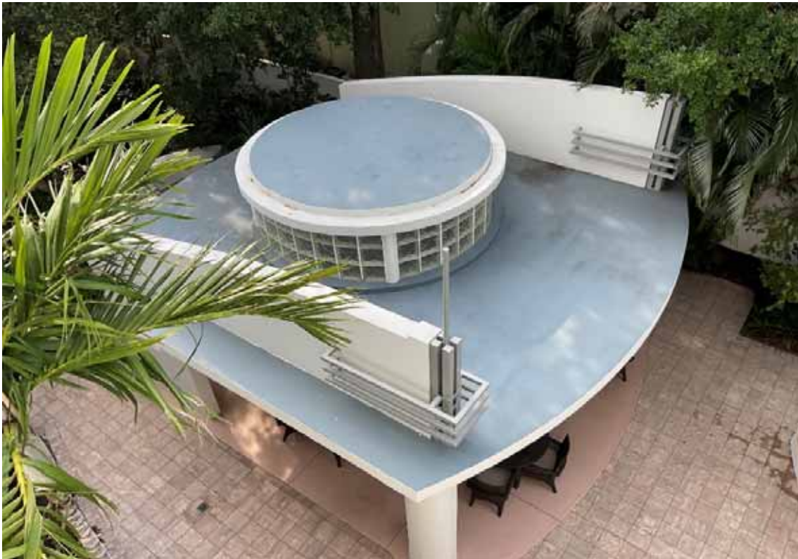
Pool Shelter Roof
